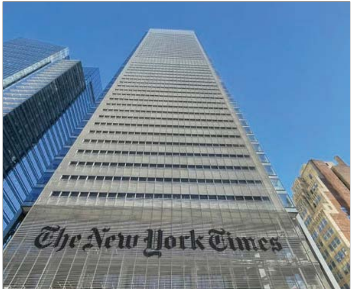
The New York Times building uses fritted glass clad with rods which make its facade more visible to birds.
